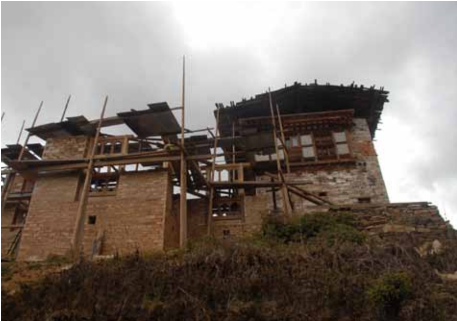
(Above) Renovations being made at the Garkhai Lhakhang (monastery) in Shingkar.
