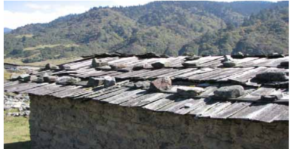
(Above) Villagers in Merak and Sakteng, two communities within the Sakteng Wildlife Sanctuary, used wood shingles for roofing.
